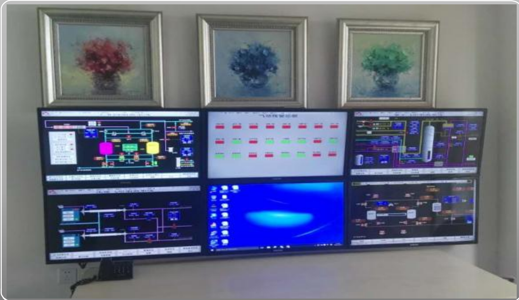
Deputy Control Centre-Shanghai China
